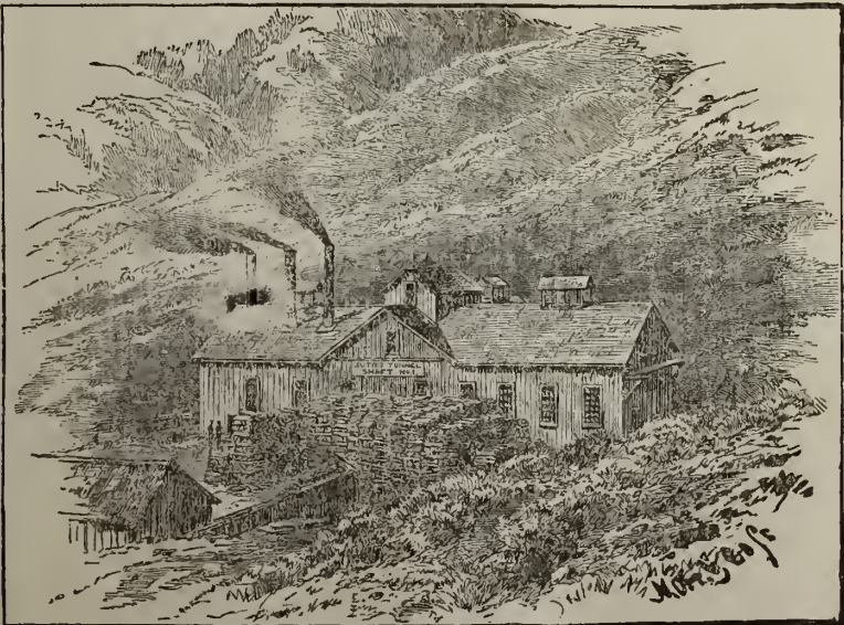
VIEW OF HOISTING WORKS AT SHAFT NO. 1, SUTRO TUNNEL.
